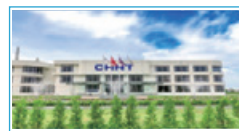
Thailand Solar Power Production Base
